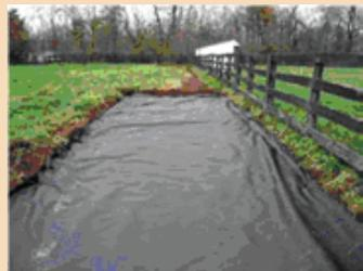
Figure 3. Geotextile fabric in place after excavation.
