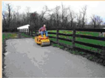
Figure 9. Compaction with drum roller.
