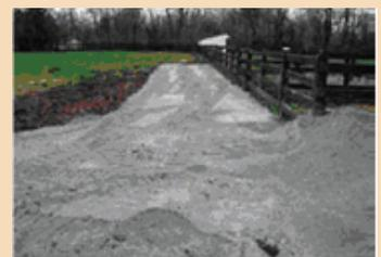
Figure 7. Surface layer of crushed stone
