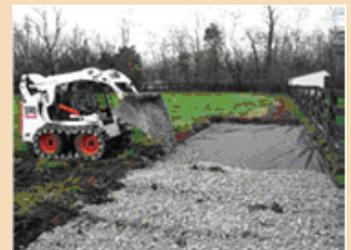
Figure 5. Base layer of crushed stone.
