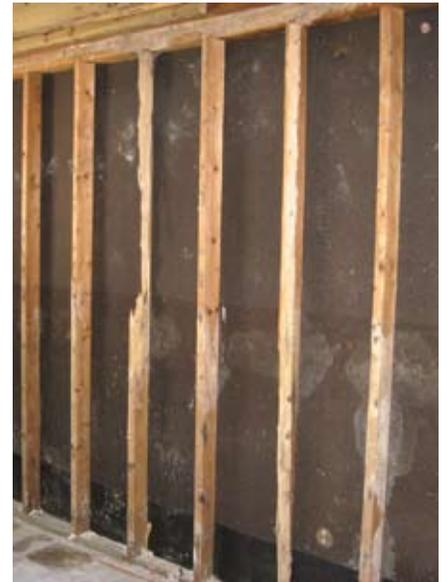
*Safety note: Walls are more vulnerable to wind when the coverings have been removed. Install temporary bracing to keep the wall from racking. Diagonal 2 x 4s work well for this.*
