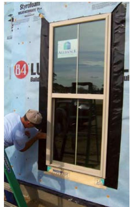
Install windows and doors so water that leaks around the frame is ushered back out. The direction of overlap and placement of tape are very important.
