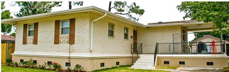
**Elevated Homes** – New homes in flood-prone areas must be elevated. This can be achieved by building the house on a raised foundation of piers, piles or foundation walls or atop a mound of structural fill dirt.
