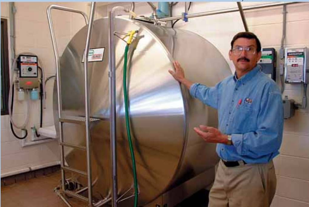
Michael E. McCormick, dairy nutrition researcher, is in the milk room in the new double-five (10 stalls) milking parlor at the Southeast Research Station. This bulk milk tank stores 3,000 gallons.
