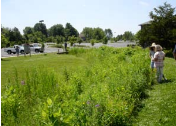
Bioretention seeding in Columbia, Missouri reduces maintenance costs associated with mowing, mulching, and weeding.
