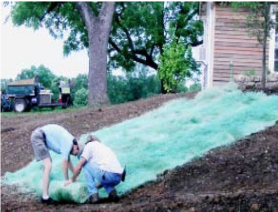
Unroll erosion control blankets from top of slope to bottom and overlap edges to attain complete coverage. Pin down blankets securely.
