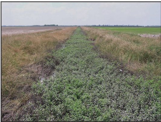
Vegetated drainage ditch
