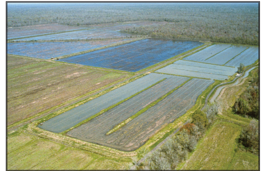
Baffle levees for water circulation
