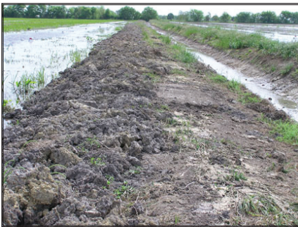
Levee re-built from sediment
