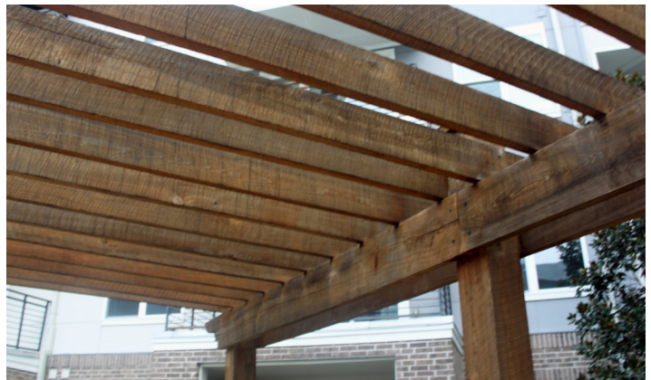
The rafters of a pergola are the component of which offers the desired shading. The spacing between the rafters and the height of each rafter help determine the amount of shading it provides.
