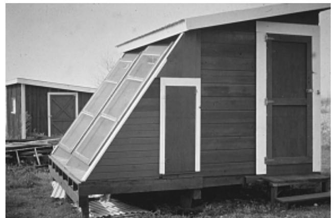
**Figure 11.** East side of solar lumber dryer showing principal loading and unloading door and the small access to collector area. (Photo courtesy of USDA Forest Products Laboratory).
