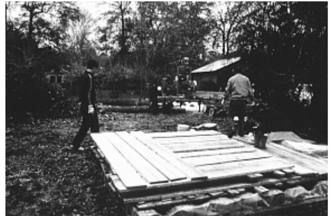
**Figure 6b.** A poor stacking job with no stickers between boards. There is little ventilation under or inside the pile. Lumber piled in this fashion may lead to warp, check, stain and decay.
