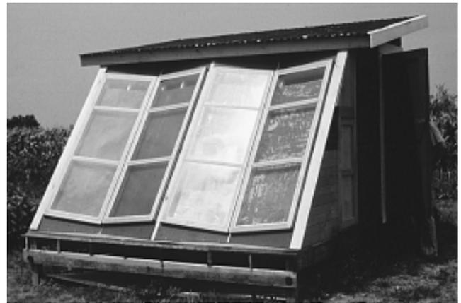
**Figure 10.** The front south side view of a solar-heated lumber dryer. (Photo courtesy of USDA Forest Products Laboratory).
