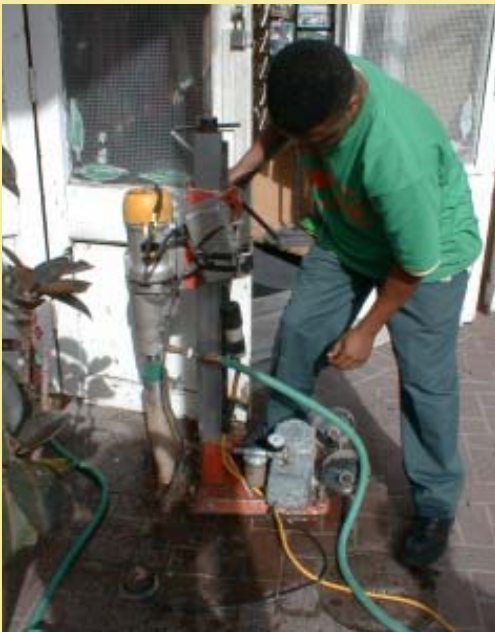
Photo 19. Drilling hole in concrete foundation to install bait station
