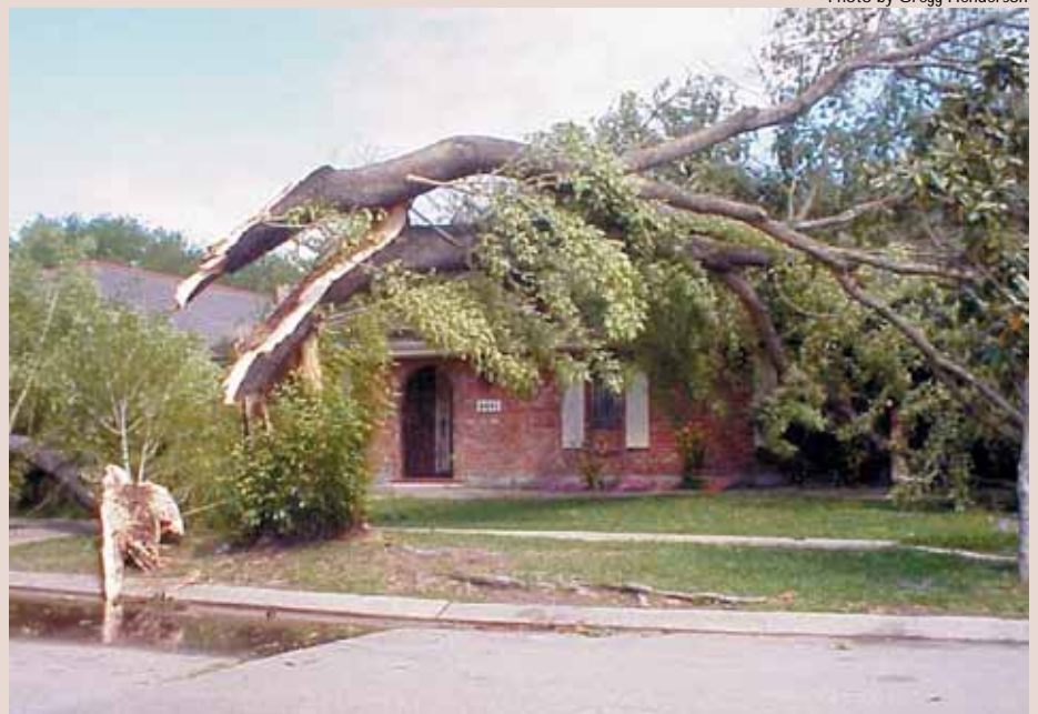
This tree was so weakened from termite infestation that high winds blew it onto this house in New Orleans.
