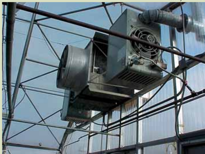
Figure 1. Traditionally, furnaces are suspended as high as 10 feet above the greenhouse ground level.
