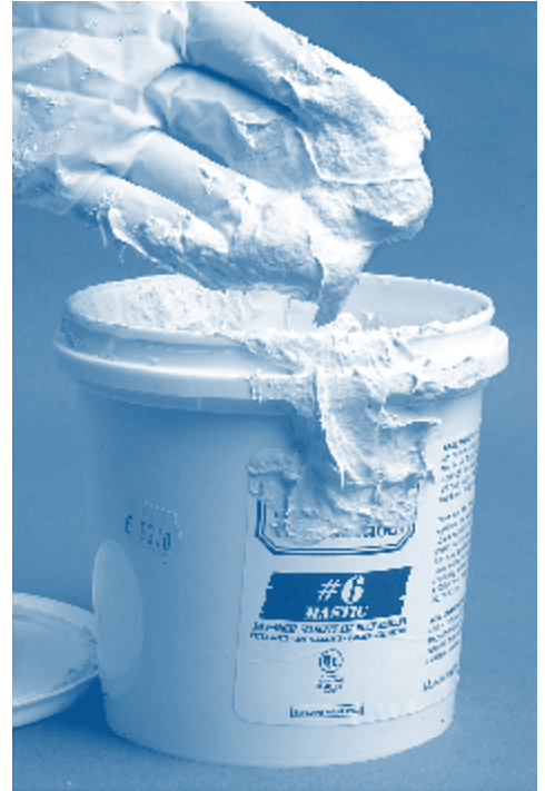
Seal air ducts with mastic
