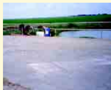
Wash pad with collection pond
