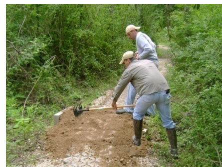
Jacob Morrison and Zachary Buck, students in Applied Environmental Management (EMS 3040), work on the erosion control and bike path improvements they helped design for the BREC Hooper Road Park as their service-learning activity.
